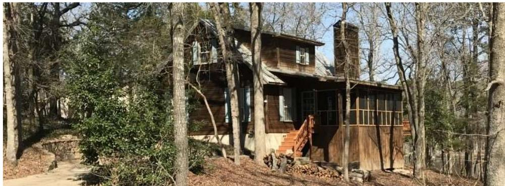
*While the fire-rated roofing material and properly pruned trees offer some protection from wildfire risk, the woodpile next to the deck and the flammable siding and skirting pose hazards.*
